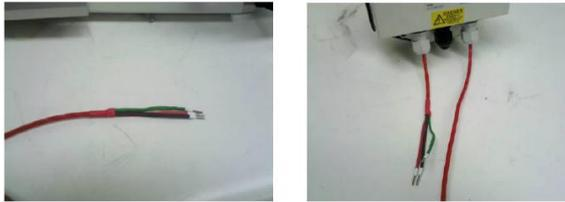
Using power and Ethernet cables that have been passed through cable glands on rear of enclosure, install cables onto camera (turn on camera if needed).
