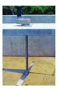
**Vertical Flocculator Shaft and Motor**
